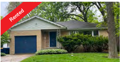
1614 Berkeley Rd. ♦ Highland Park $3,500 *Represented the Tenants
